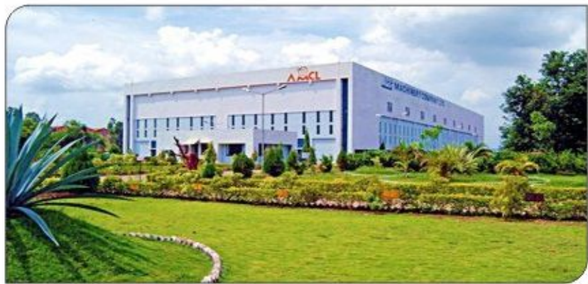
Works at Nagpur
