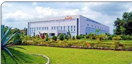
works at nagpur
