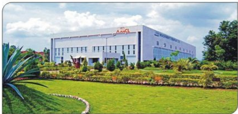
Works at Nagpur
